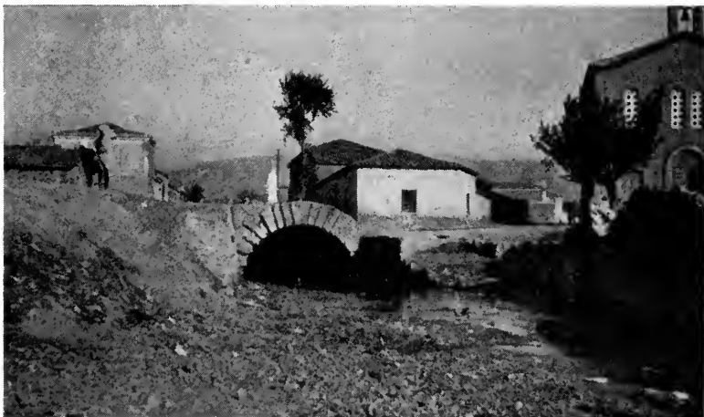
AN OUTFALL SEWER NEAR DANIELS' CHURCH, ATHENS
